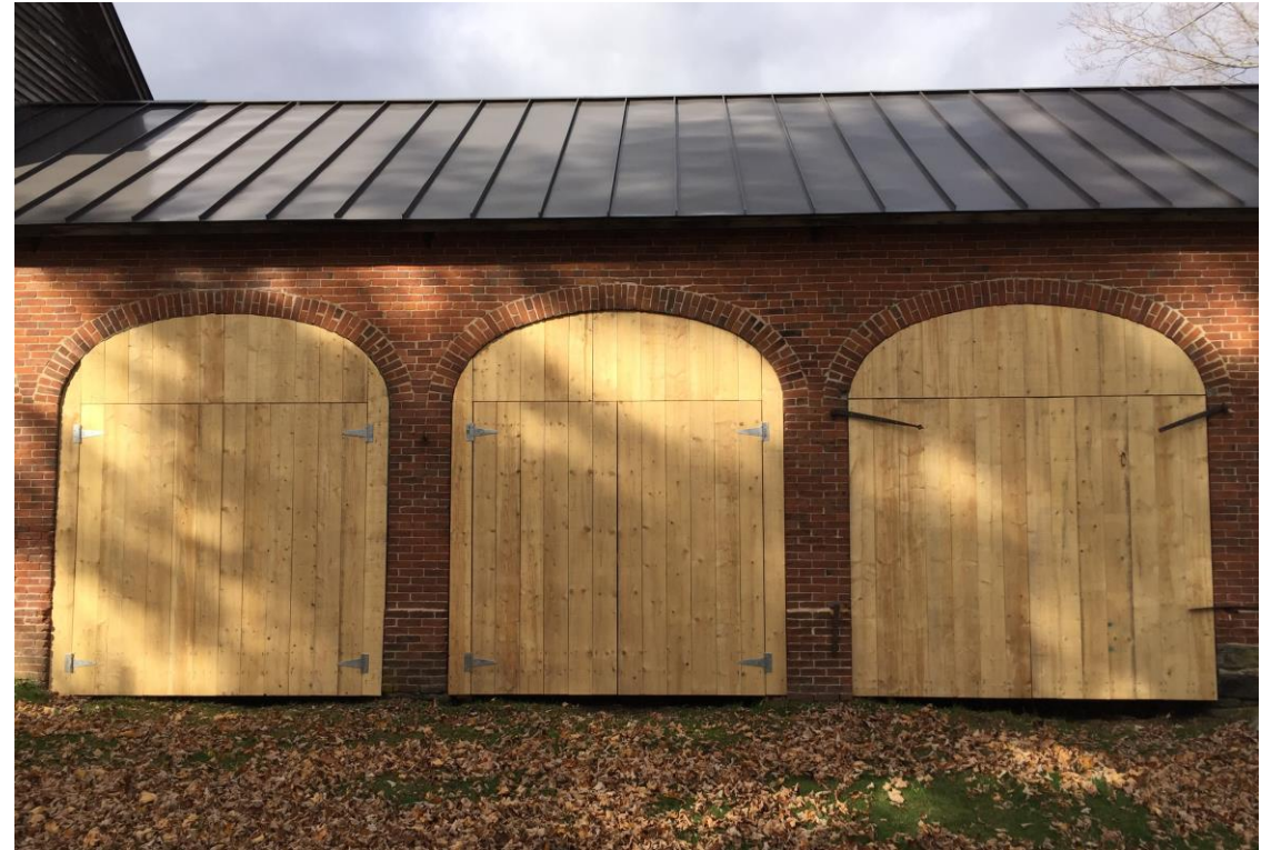
Replicated severely deteriorate doors and hinges
