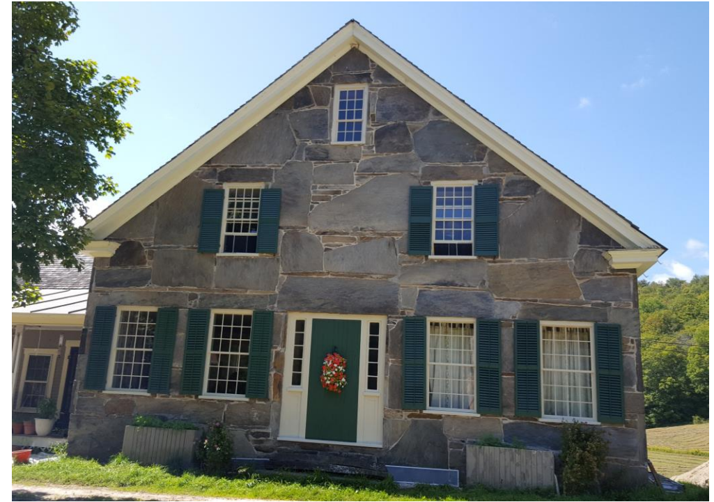
Replicated missing windows and restored original sash
